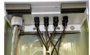
Detail of the cable feed-through on the bottom of the enclosure
